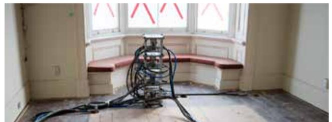
Proprietary, high performance, low volume grout pumps deliver cementitious grout to a multitude of grout monitors, set up in injection circuits. Each monitor operates up to 8 injection ports.
